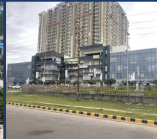
Park Town Complex
